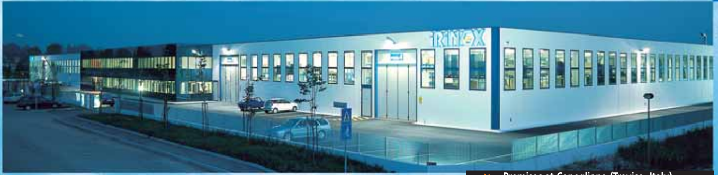
★ Premises at Conegliano (Treviso, Italy)
